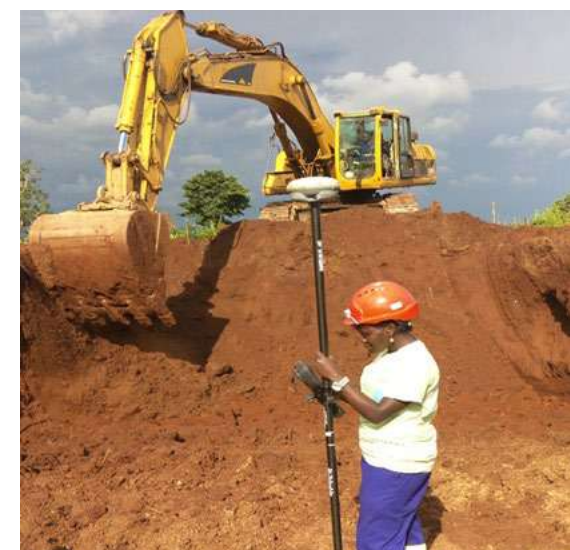
Figure 4: Surveyor setting out the mine plan at Namekara vermiculite mine
